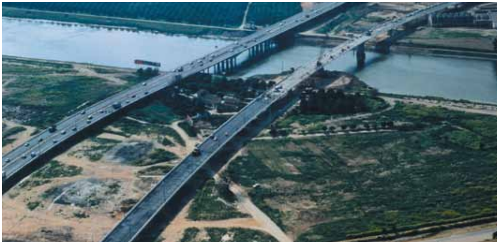
New motorway, Comunidad Valenciana, Spain. Co-financed by ERDF.
