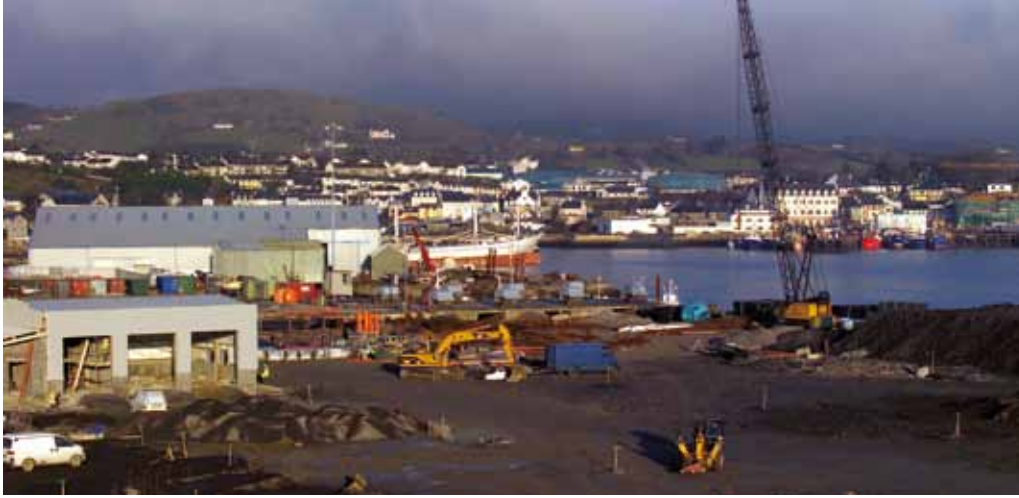
Killybegs Harbour Development, Co. Donegal, Ireland
