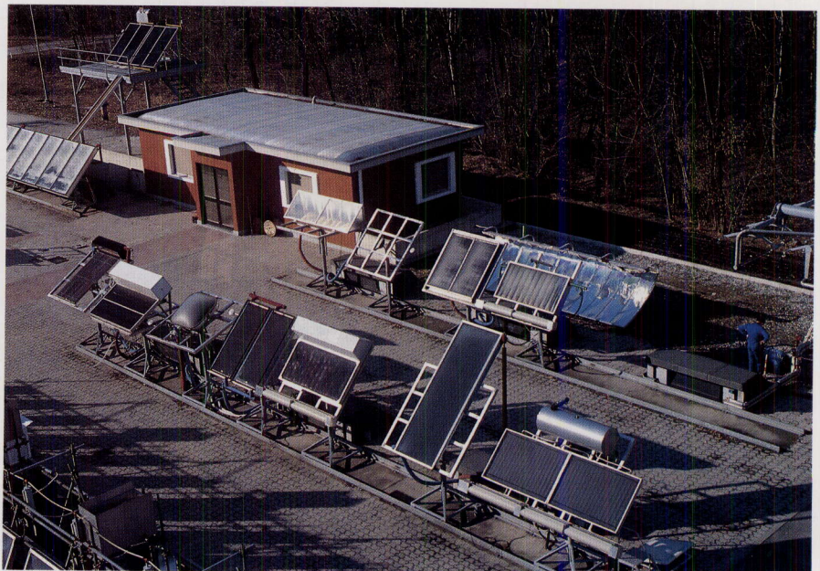
Figure 67: 11 different commercial Solar water heating Systems under test as part of an activity for the development of a test procedure in determining the long term thermal performance
