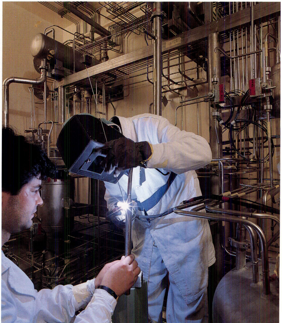
Figure 88: Completing work inside one of the PETRA experimental cells
