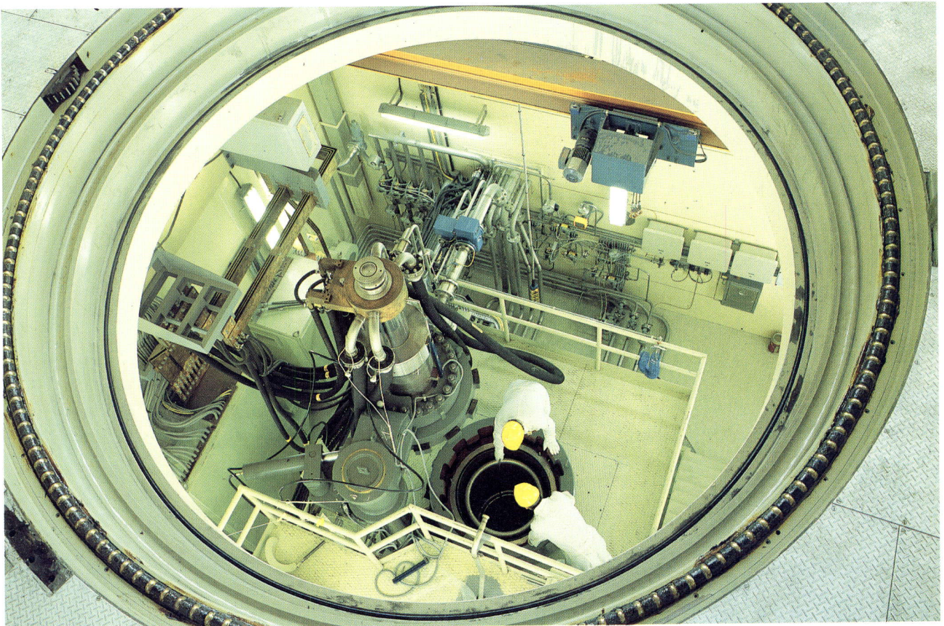
Figure 82: A 'birds-eye' view of the FARO facility showing preparational work on the UO 2 melting furnace
