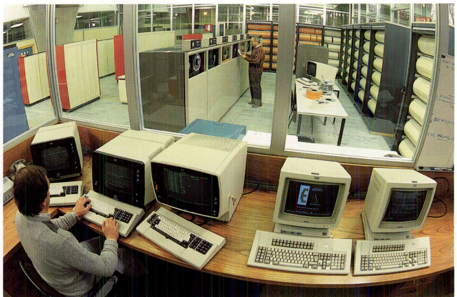
Figure 52: View of the mainframe computing system from the operators' control room
