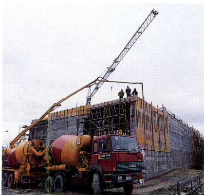
Figure 56: The ETHEL Laboratory in an advanced stage of construction.
