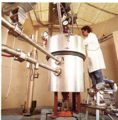
Installation of the 100 liter chemical batch reactor within the FIRES bunker
