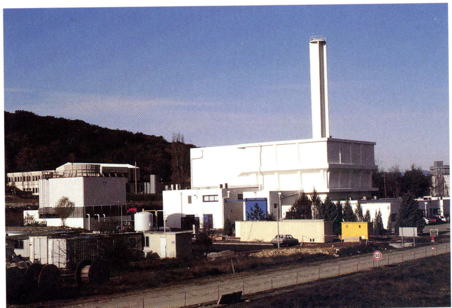
External view of the PHEBUS complex at the CEN Cadarache
