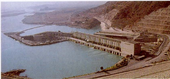
Building a large dam is indispensable for better water management, but it is expensive and usually requires assistance from many donors
