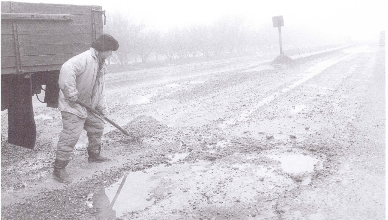
Maintenance works on the Tashkent to Samarkand road
