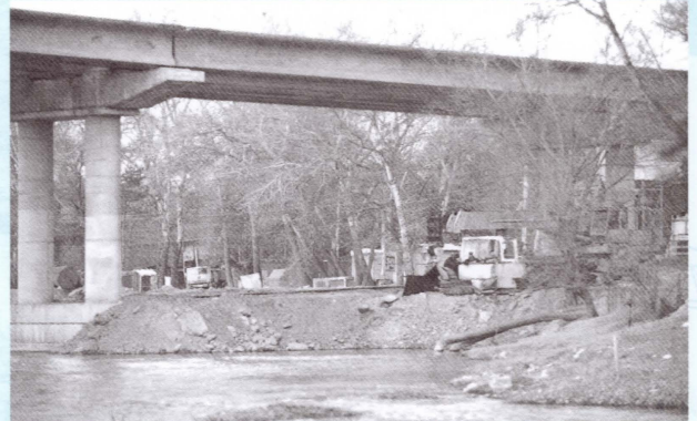
Construction of a new Red Bridge between Georgia and Azerbaijan
