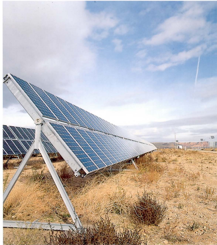
The 1MW photovoltaic plant established outside of Toledo, Spain, uses both mono- and polycrystalline cells (left and right, respectively).
