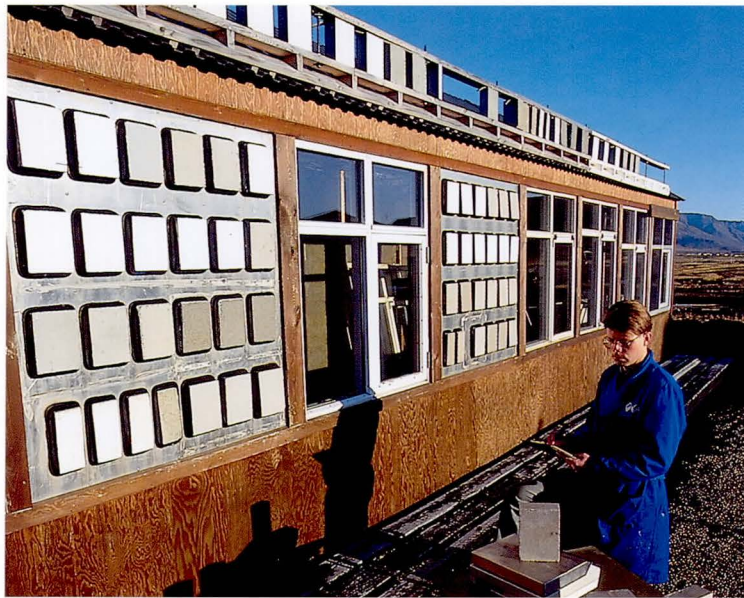
Various concrete coatings were also tested outside.
