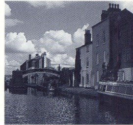
Gas Street Basin, canal development - Birmingham
