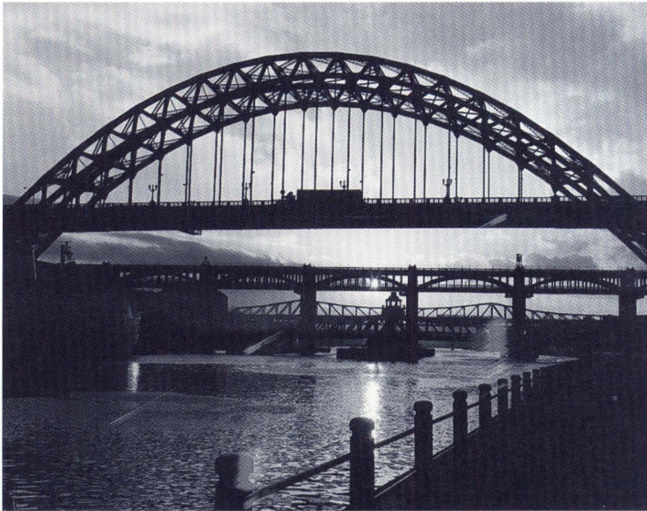
Bridges over the River Tyne - Newcastle
