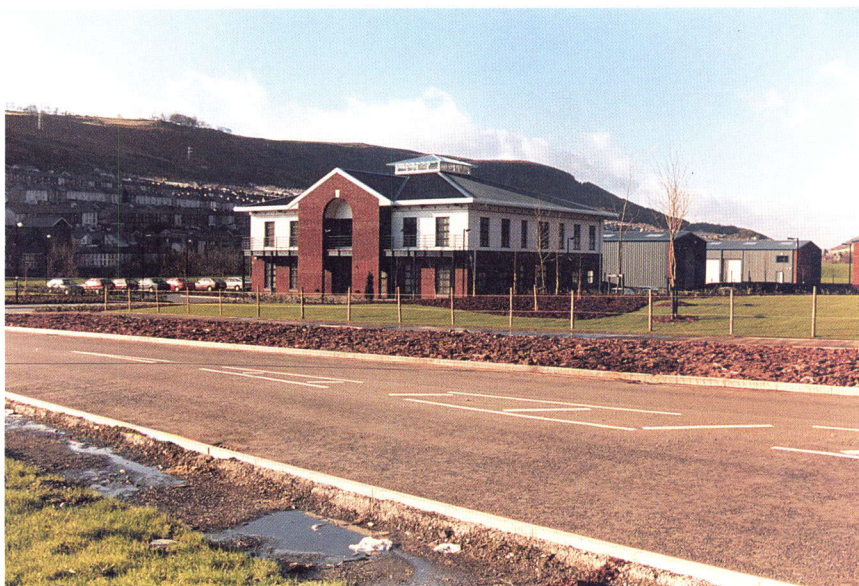
Cwm Cynon Business Centre, Aberdare.
