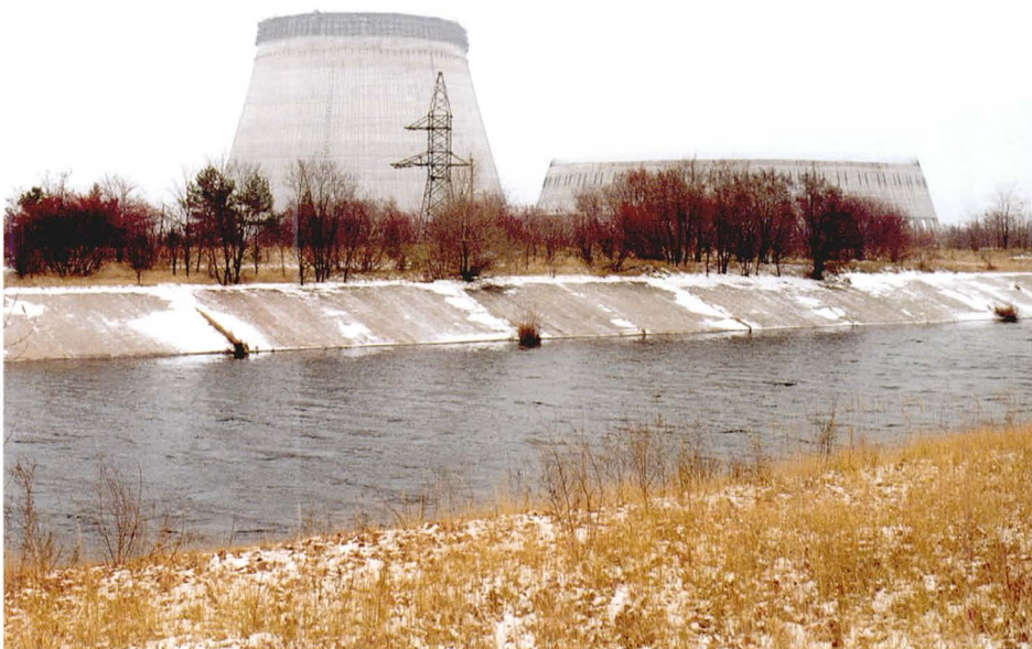
Chernobyl Nuclear Power Plant. One of the cooling towers under construction at the time of the accident; now shut down.
