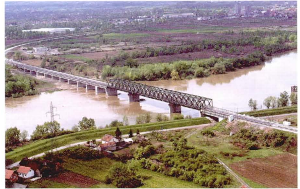
Samac Bridge reconstructed.
