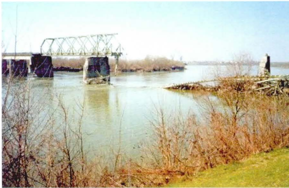
Samac Bridge before reconstruction.
