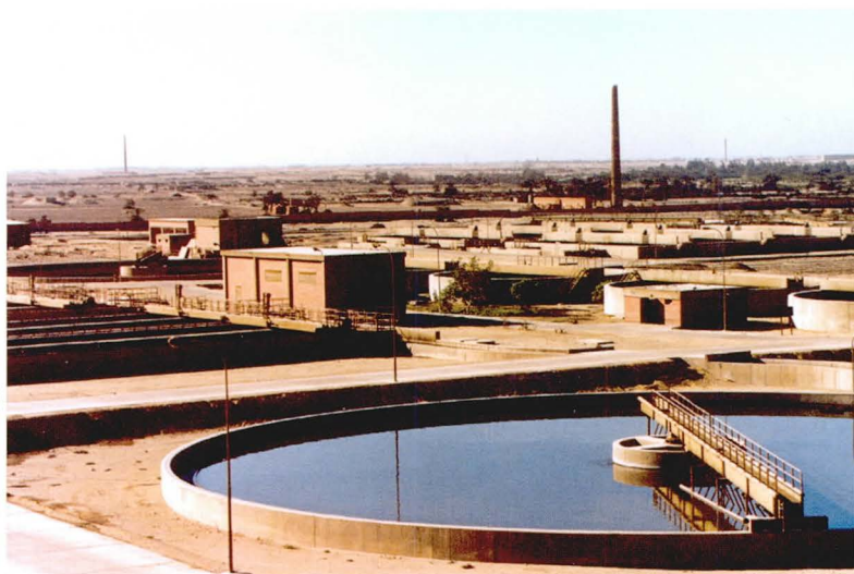
Helwan wastewater project in Helwan district (Egypt).
