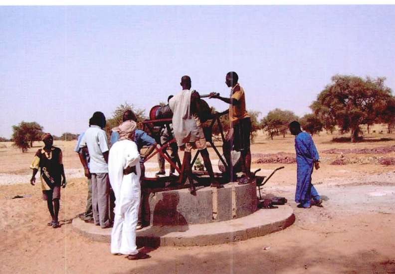
Building a well in northern Niger.
