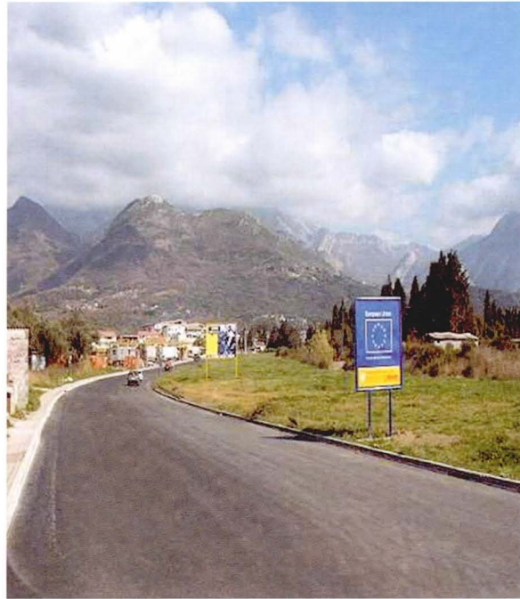
Rehabilitated road section — Podgorica to Bar (Montenegro).
