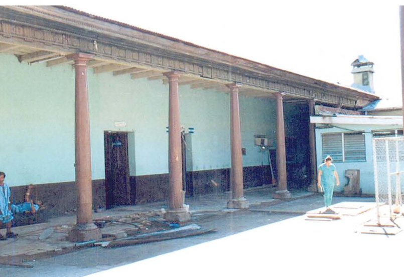
Sonsonate hospital in El Salvador before rehabilitation
