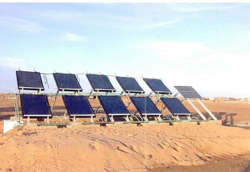
Gulf of Aqaba: desalination plant
