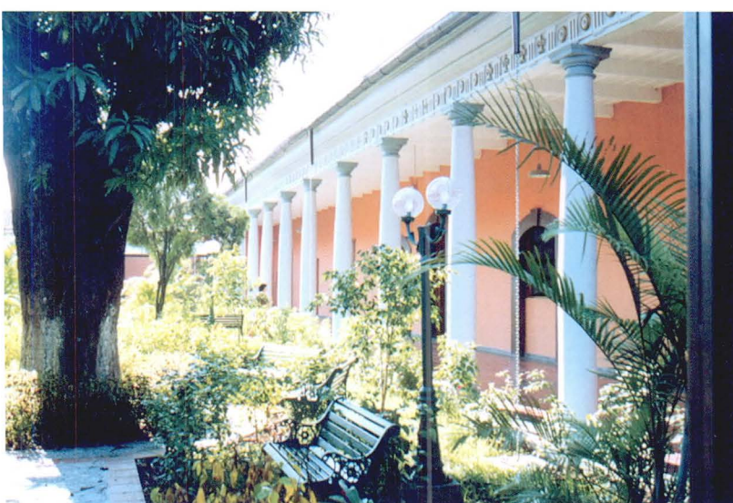
Sonsonate hospital in El Salvador after rehabilitation
