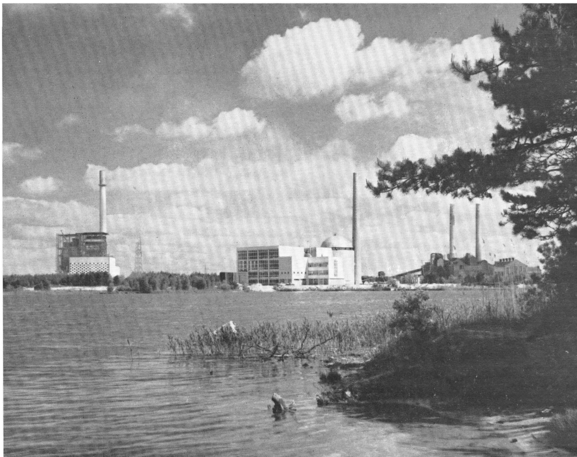
MOL (Belgium) — THE EXPERIMENTAL POWER REACTOR BR 3
