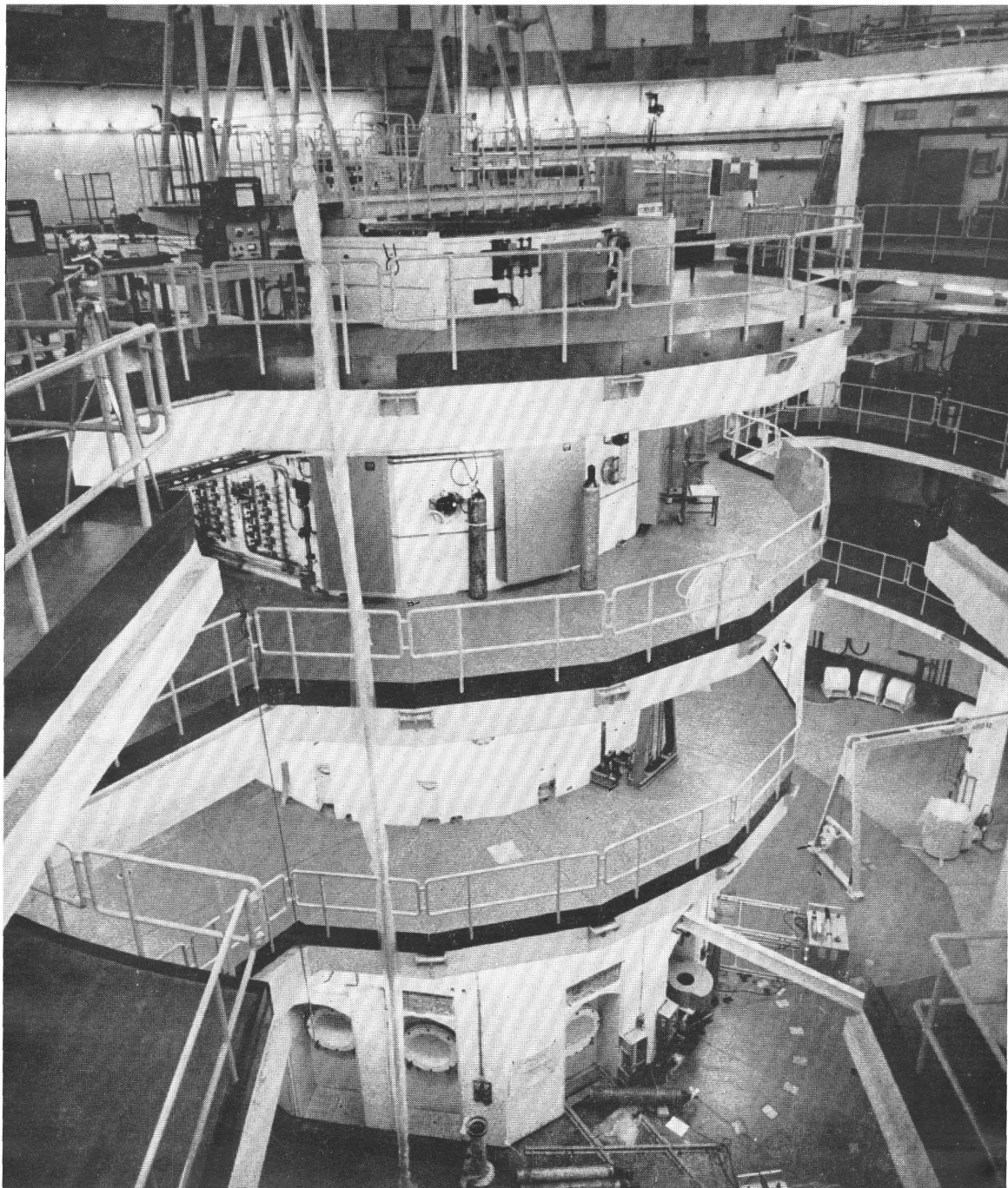
MOL (Belgium) — GENERAL OF THE BR 2 MATERIALS-TESTING REACTOR
