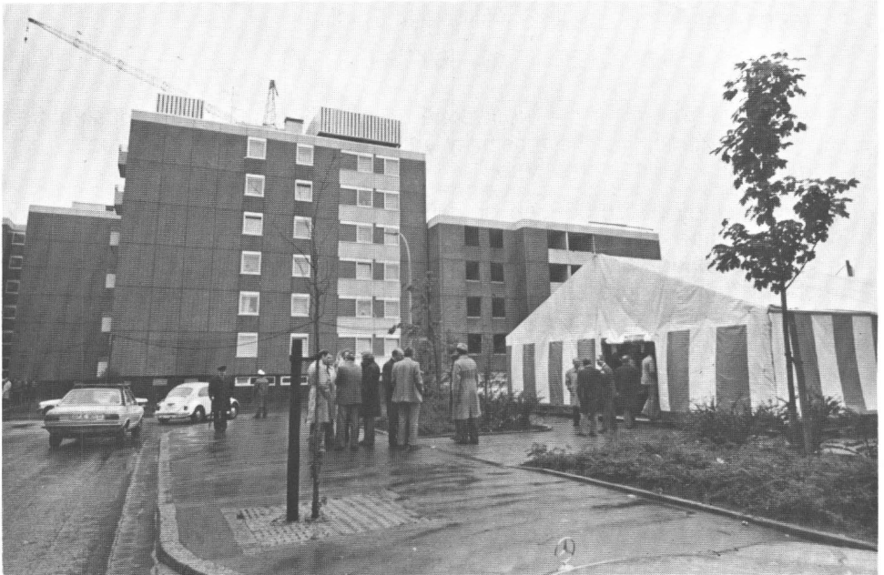
Figure 2.18.2 Apartment building heated with gas engine driven heat pump (with heat pump and heat exchangers on the roof)
