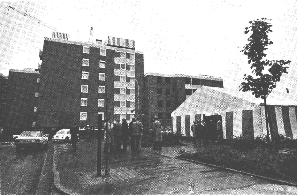
Figure 2.18.2 Apartment building heated with gas engine driven heat pump (with heat pump and heat exchangers on the roof)
