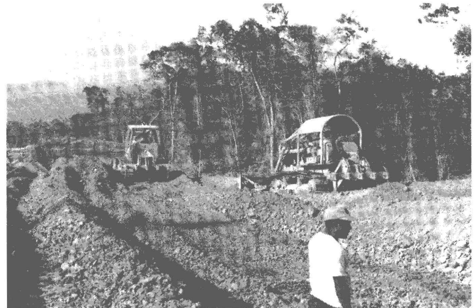
Hiritano Highway under construction.
