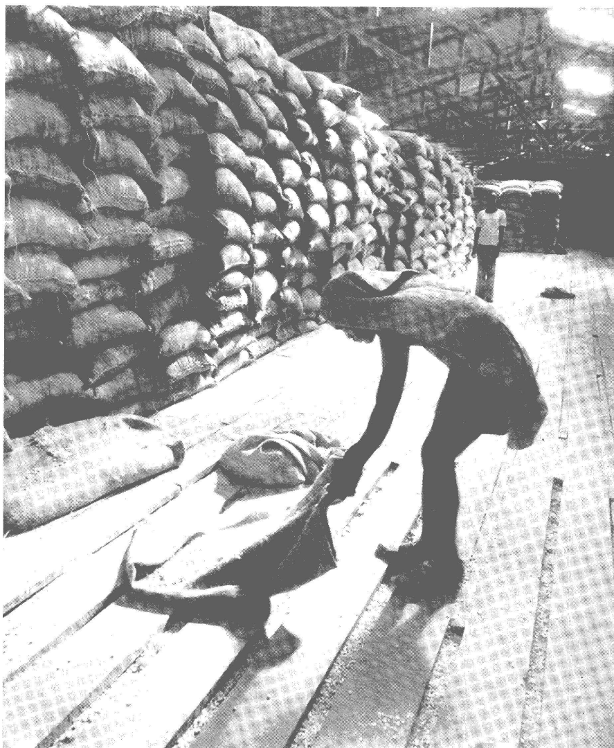
EEC-financed food store in Lodwar, Turkana district, specially built to hold food aid (photo Gartung).
