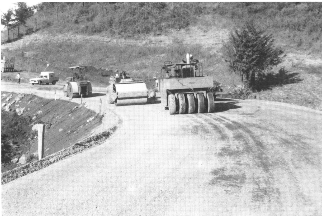
Work in progress on the Sergoit-Tambach road.
