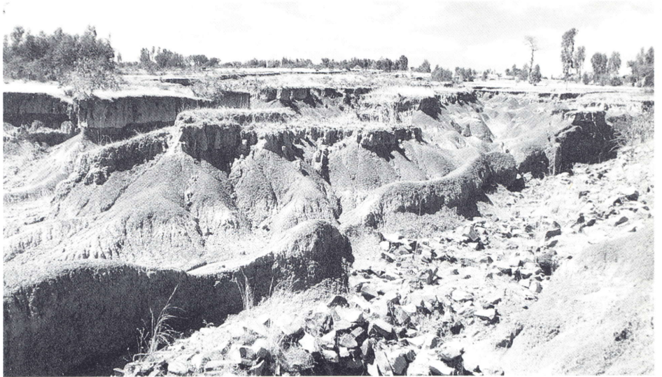
Severe erosion in South Shewa. (Photo : Tefera Zewdie)
