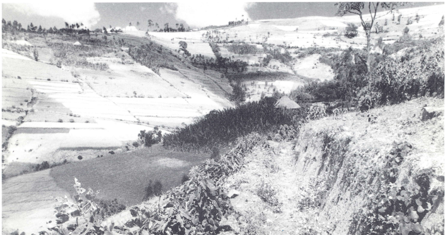
A cut-off drain in South Shewa - one of a number of techniques that help to check the formidable erosive power of run-off water. (Photo : Tefera Zewdie)
