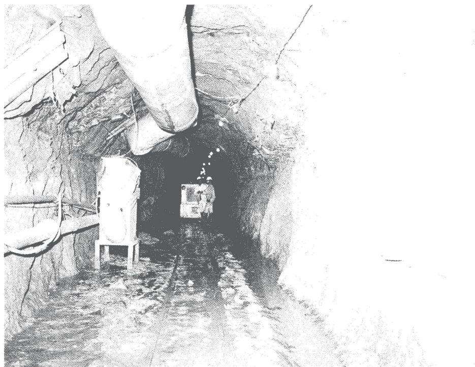
Amarti Hydropower Scheme : water diversion tunnel under construction.
