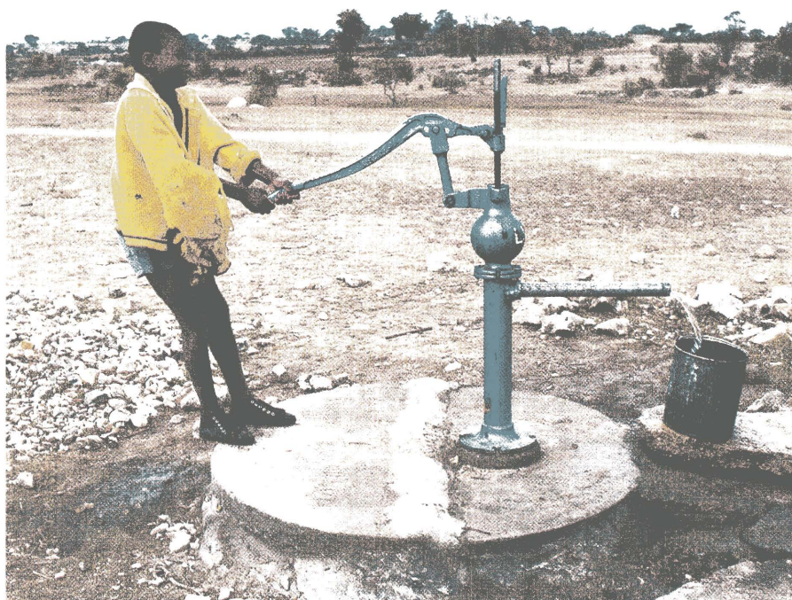
The Gokwe Rural Water Supply and Sanitation Project, when completed, should ensure that over 200,000 people will have access to clean water and sanitation
