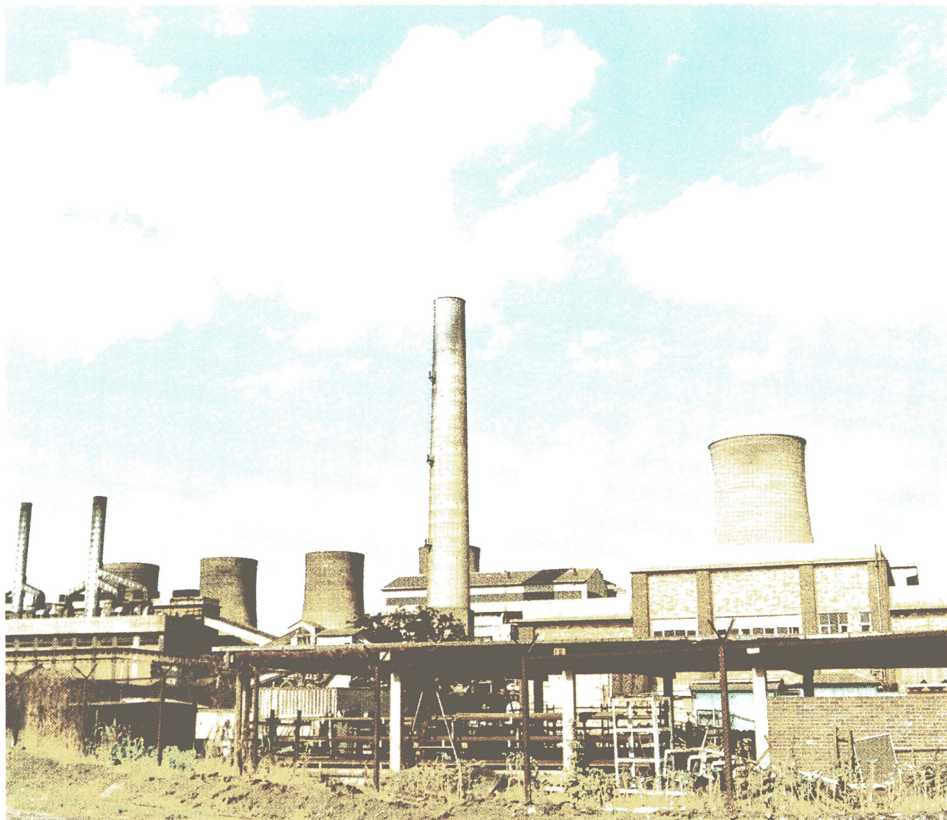
Thermal power station in Harare. Energy receives support from EIB funds
