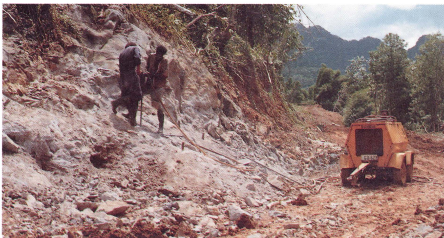
Blasting rocky terrain for a country road on Viti Levu.
