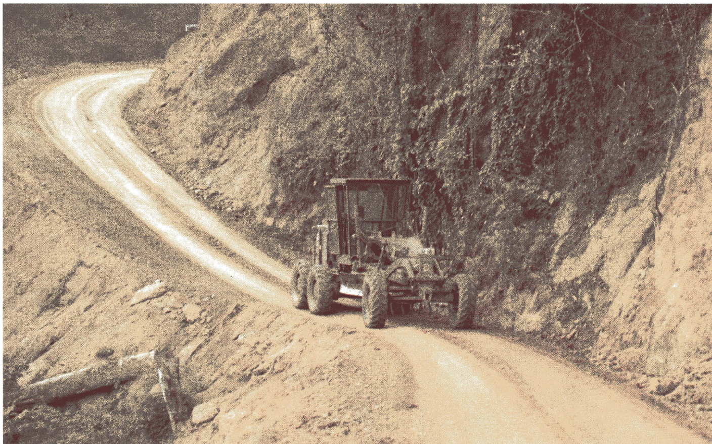
Road construction in typical rugged terrain.
