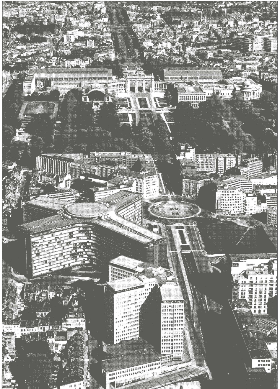
The headquarters of the Council and the Commission of the European Communities, Brussels, Belgium. (Photo : EC Commission).
