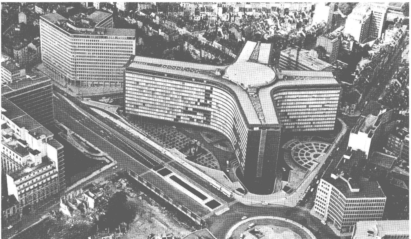
Headquarters of the Commission (centre) and the Council of Ministers (left), Brussels, Belgium.
