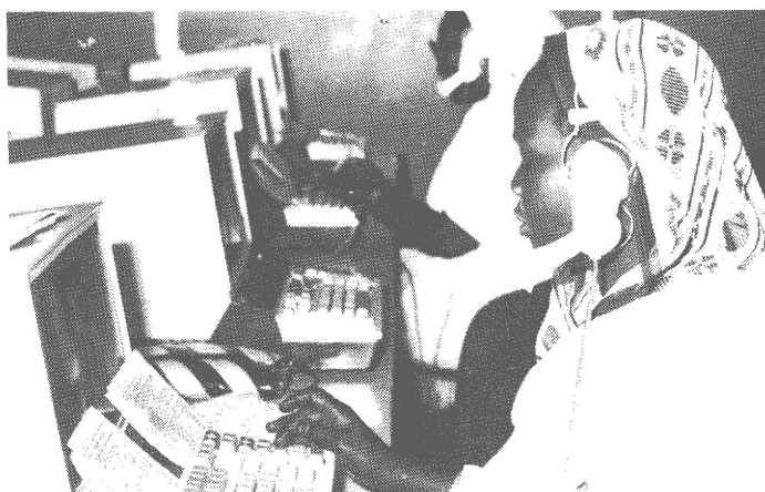
Equipment in use at the International Telephone Exchange, Khartoum.
