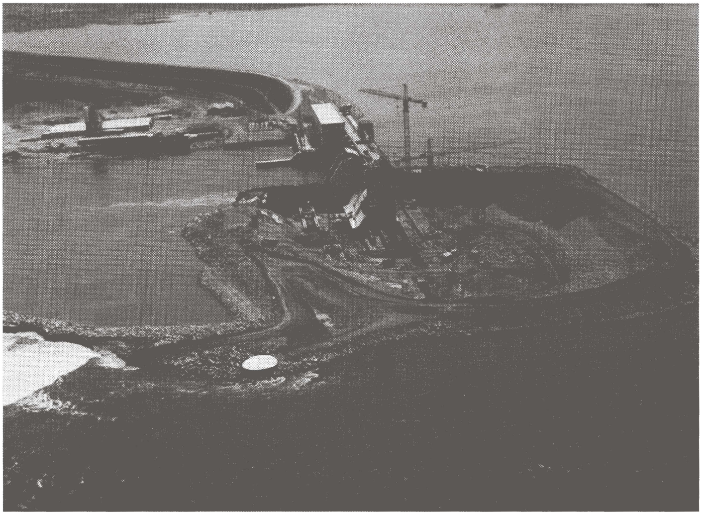
Construction of the Sélingué Dam (Mali)
