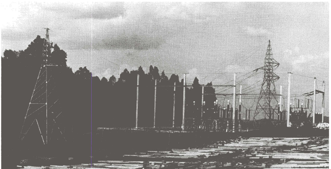
Construction of electric transmission lines in Rwanda.
