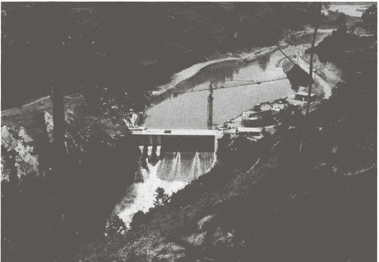
Hydroelectric power stations: EDEA 3 - Cameroon (top) Mukungwa - Rwanda (bottom)
