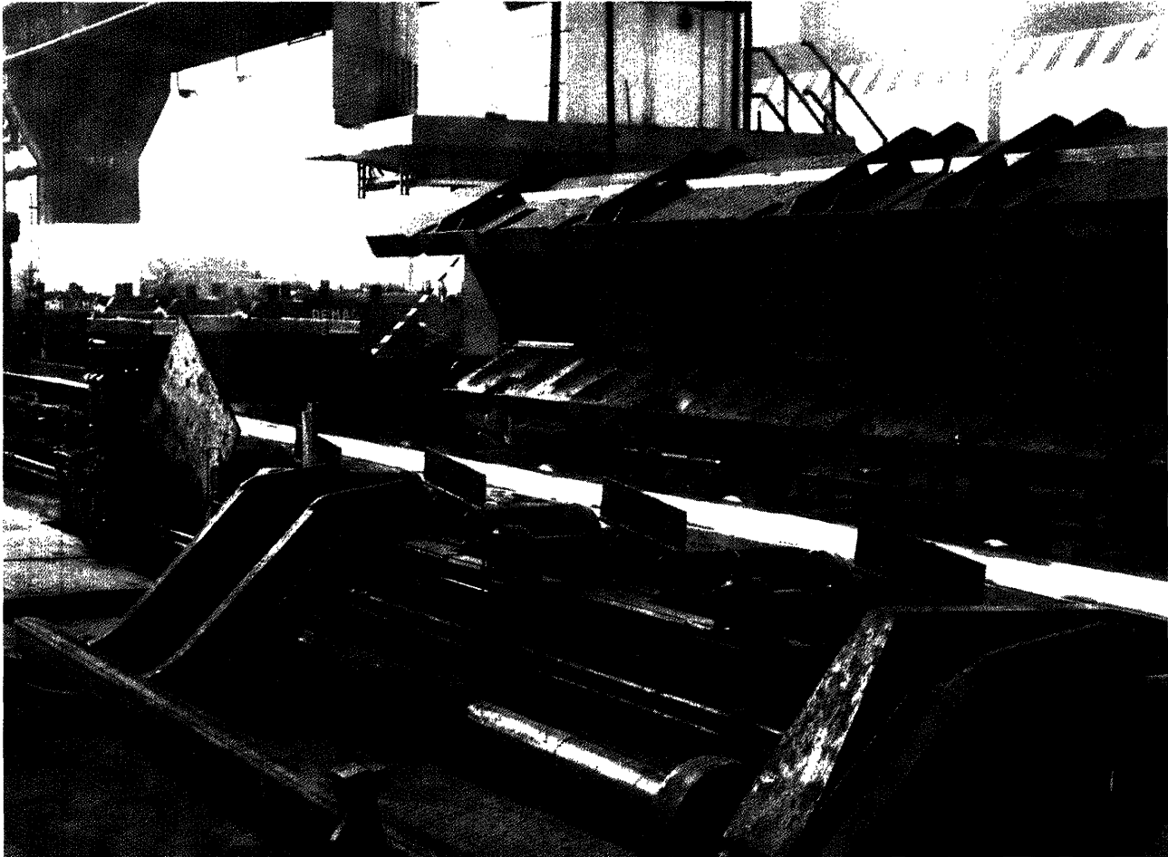
Continuous rolling mill: roller bed upstream of No 1 stand (SMS).
