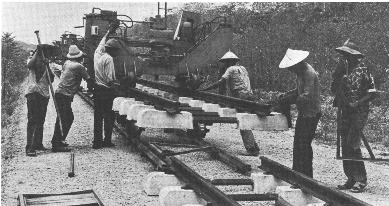
Works on the railway connection Agboville-Dimbokro
