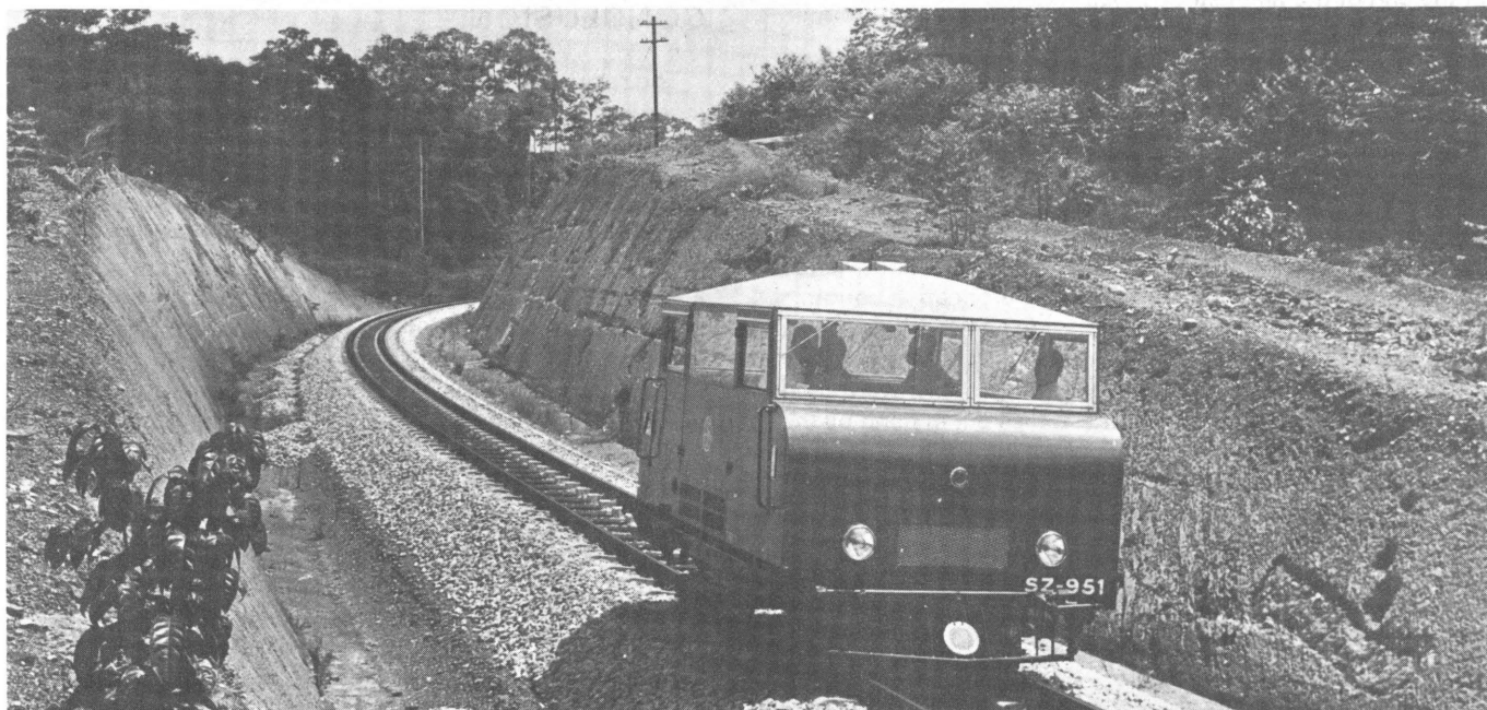
New railway connection Agboville-Dimbokro
