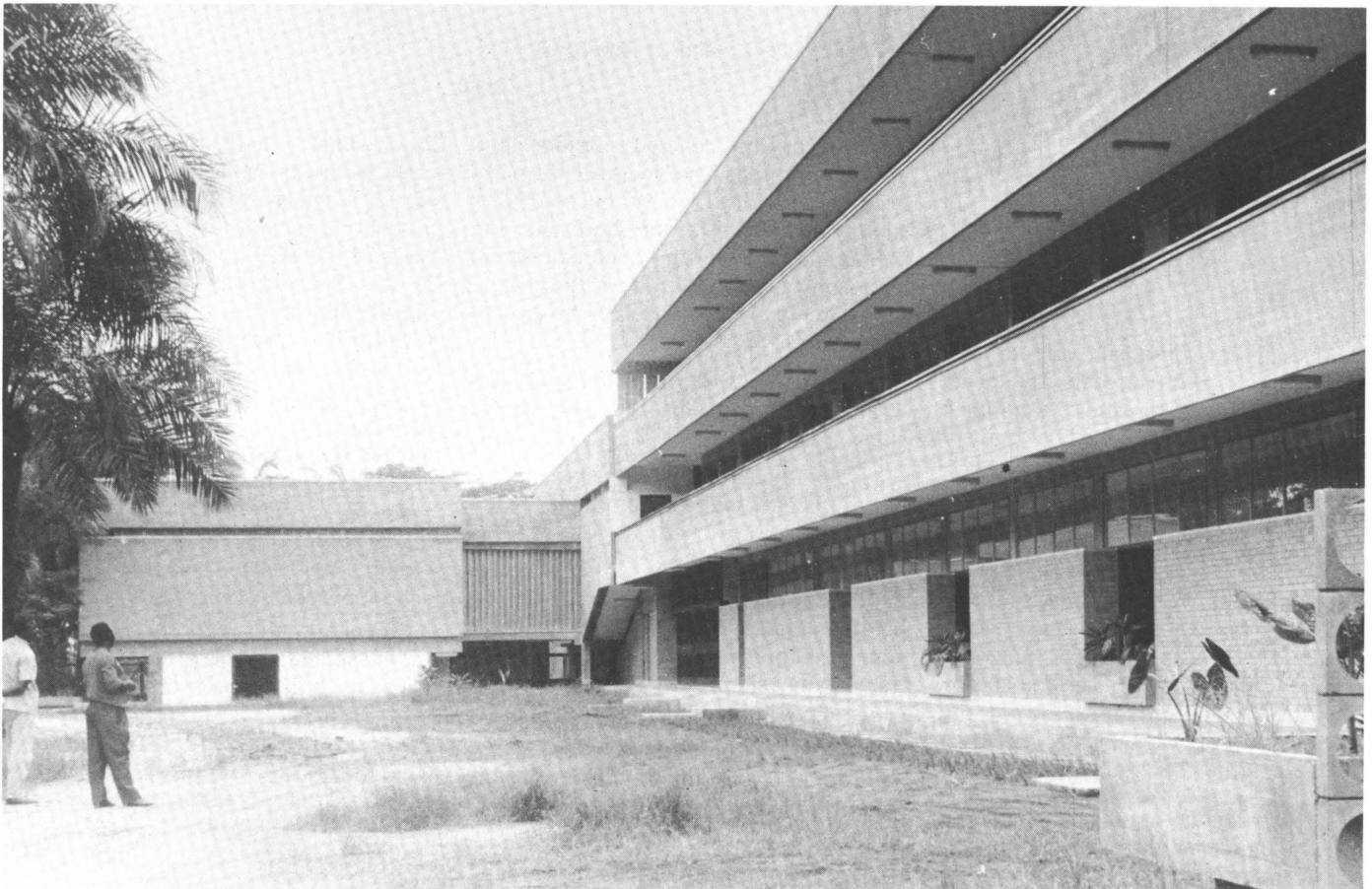
Kinshasa-Gombe High School: classrooms
