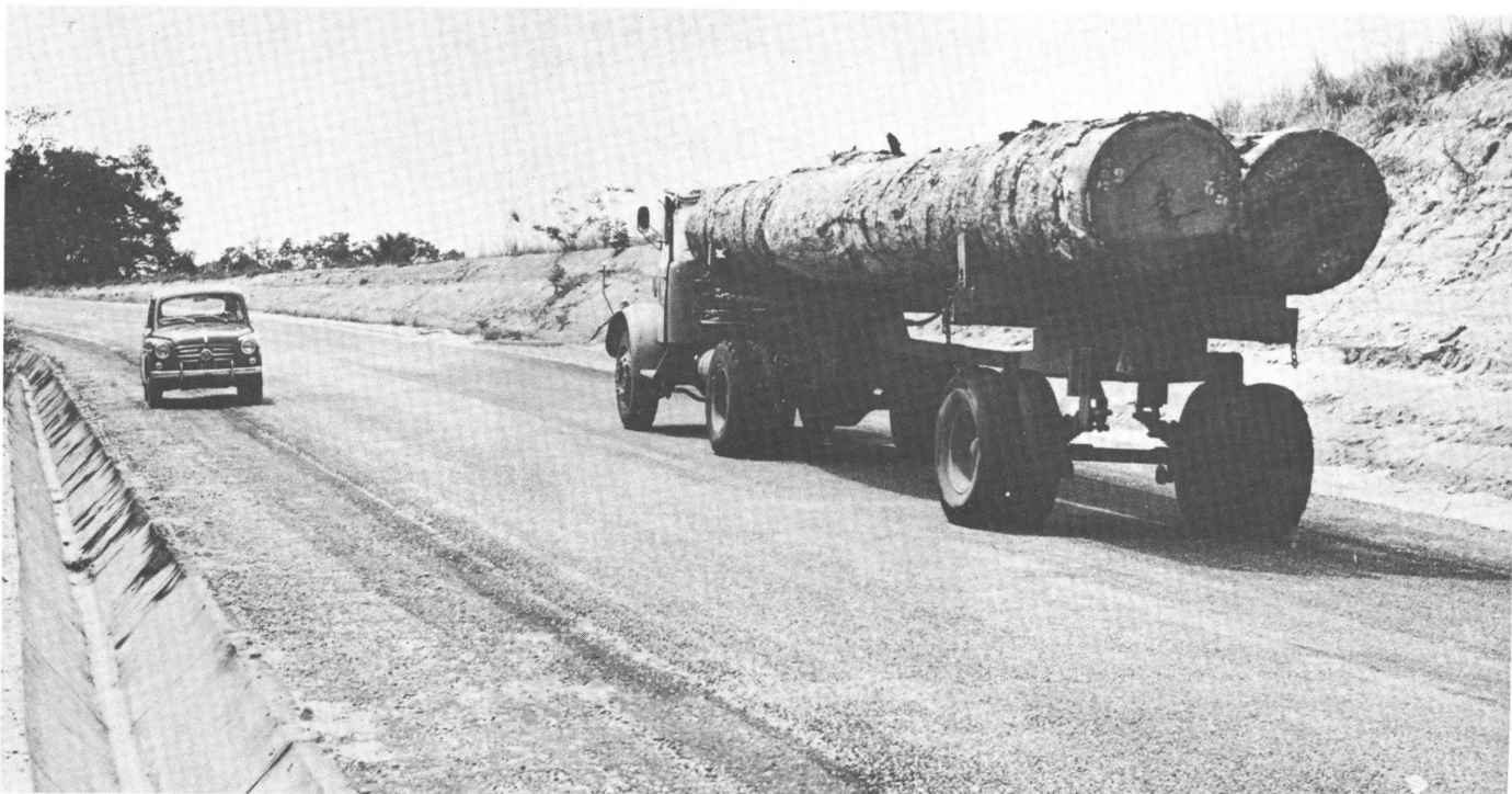
Roads and trucks for carrying timber (Congo)
