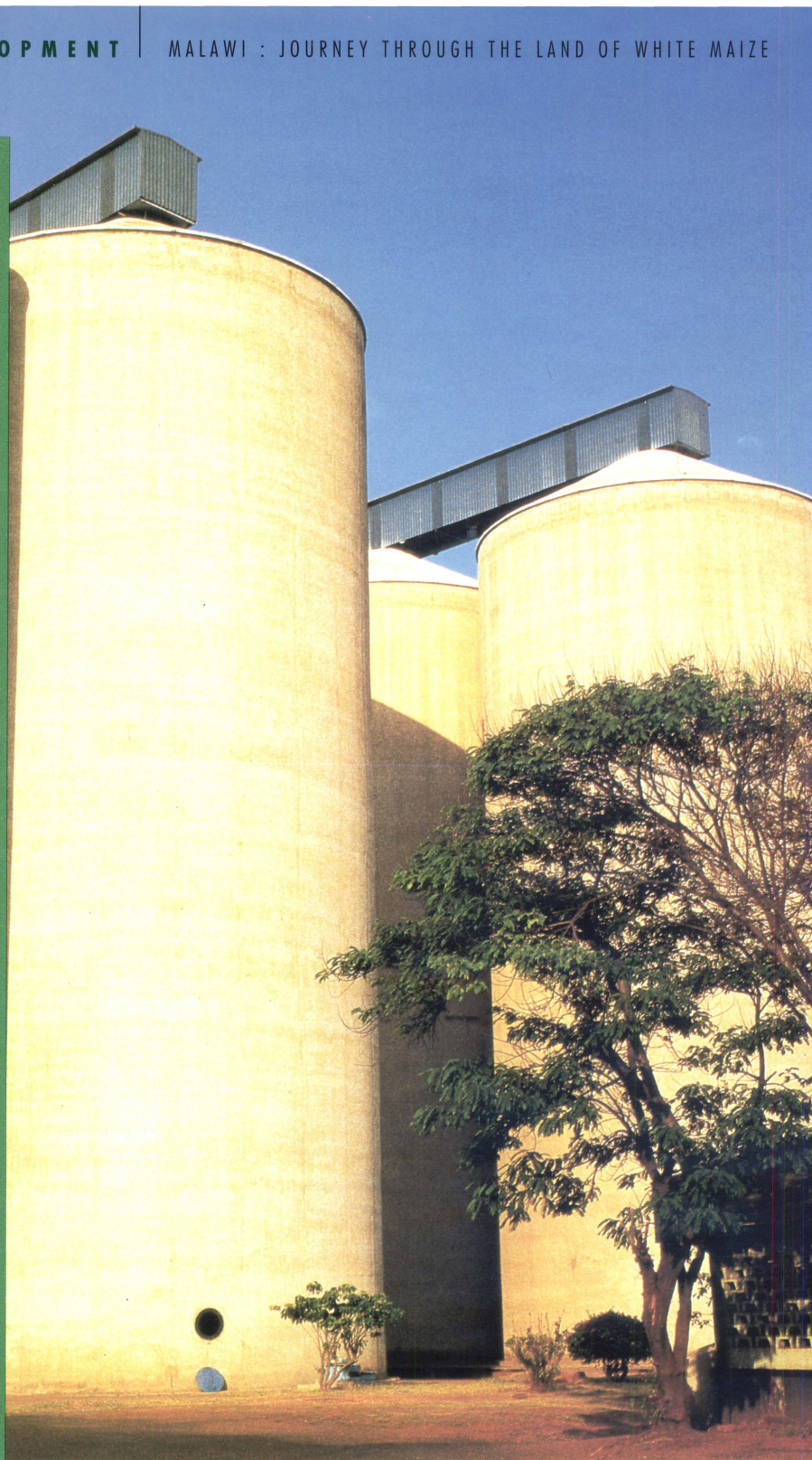
Partial view of the storage infrastructure of the ADMARC's national strategic cereal reserve in Lilongwe.
