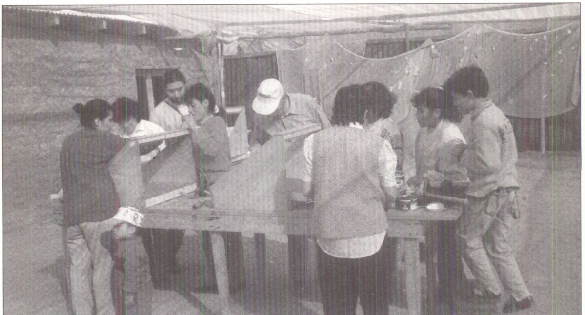
Construction of solar ovens to maximise energy efficiency, Chile
