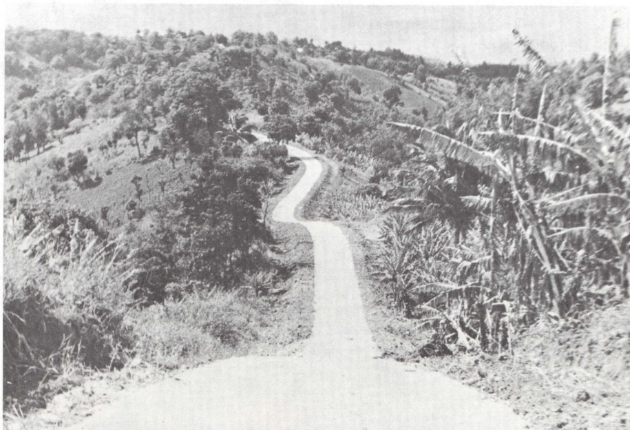
Building the access road on the Leeward Coast (Côte Sous-le-Vent), Guadeloupe.
