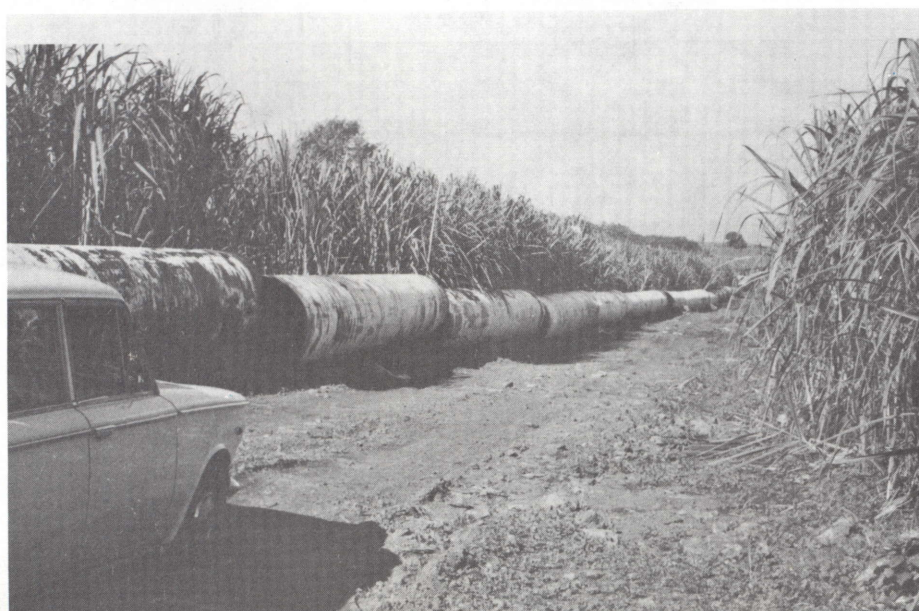
Laying the main pipe, Bras de la Plaine.
