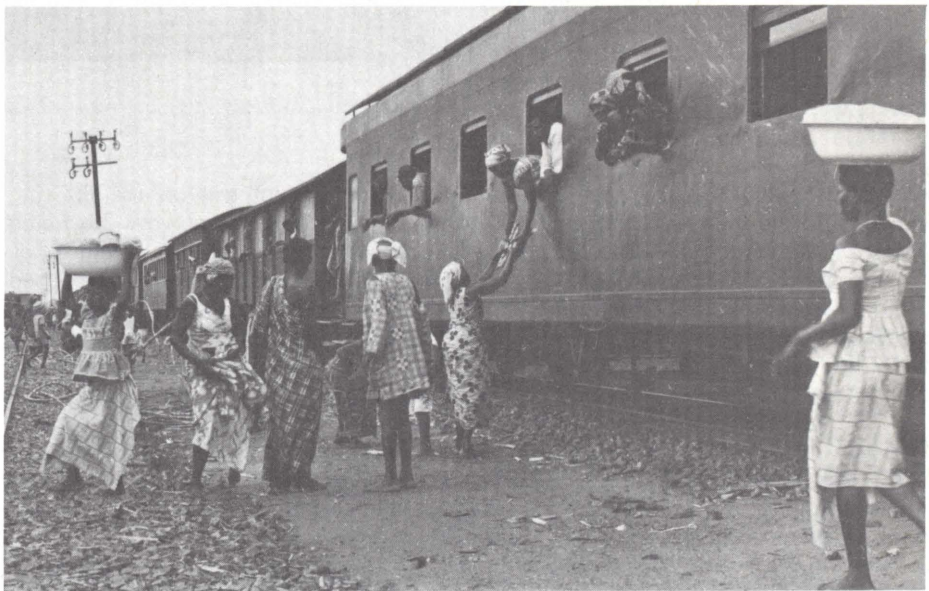
Passenger train in Tsévié station.
