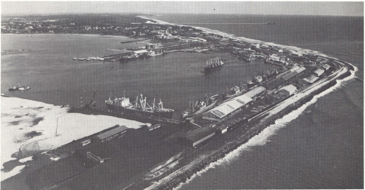
Port at Pointe-Noire (Congo), general view.
