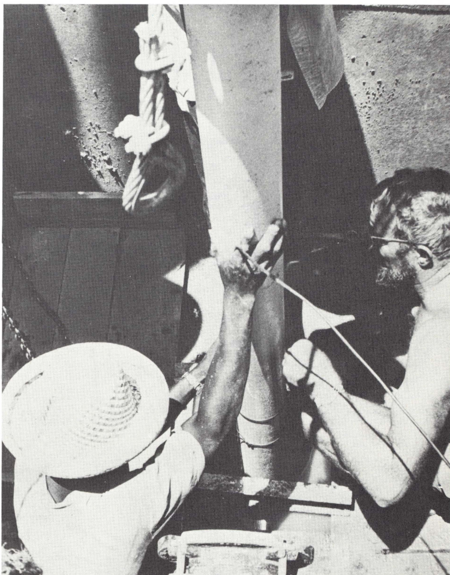
Drilling for water and pipe-laying in Guadeloupe.
