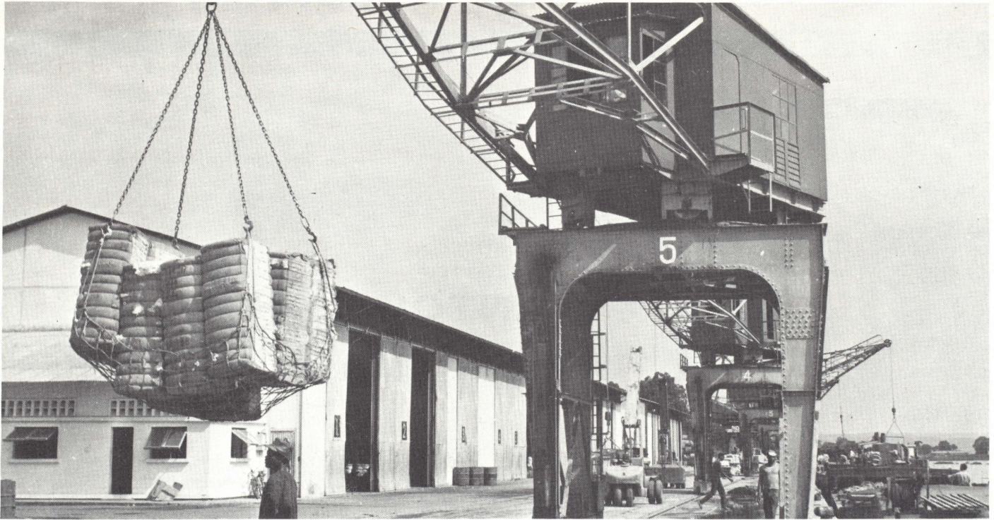
Cranes in the port of Pointe Noire (Congo Rep.)
