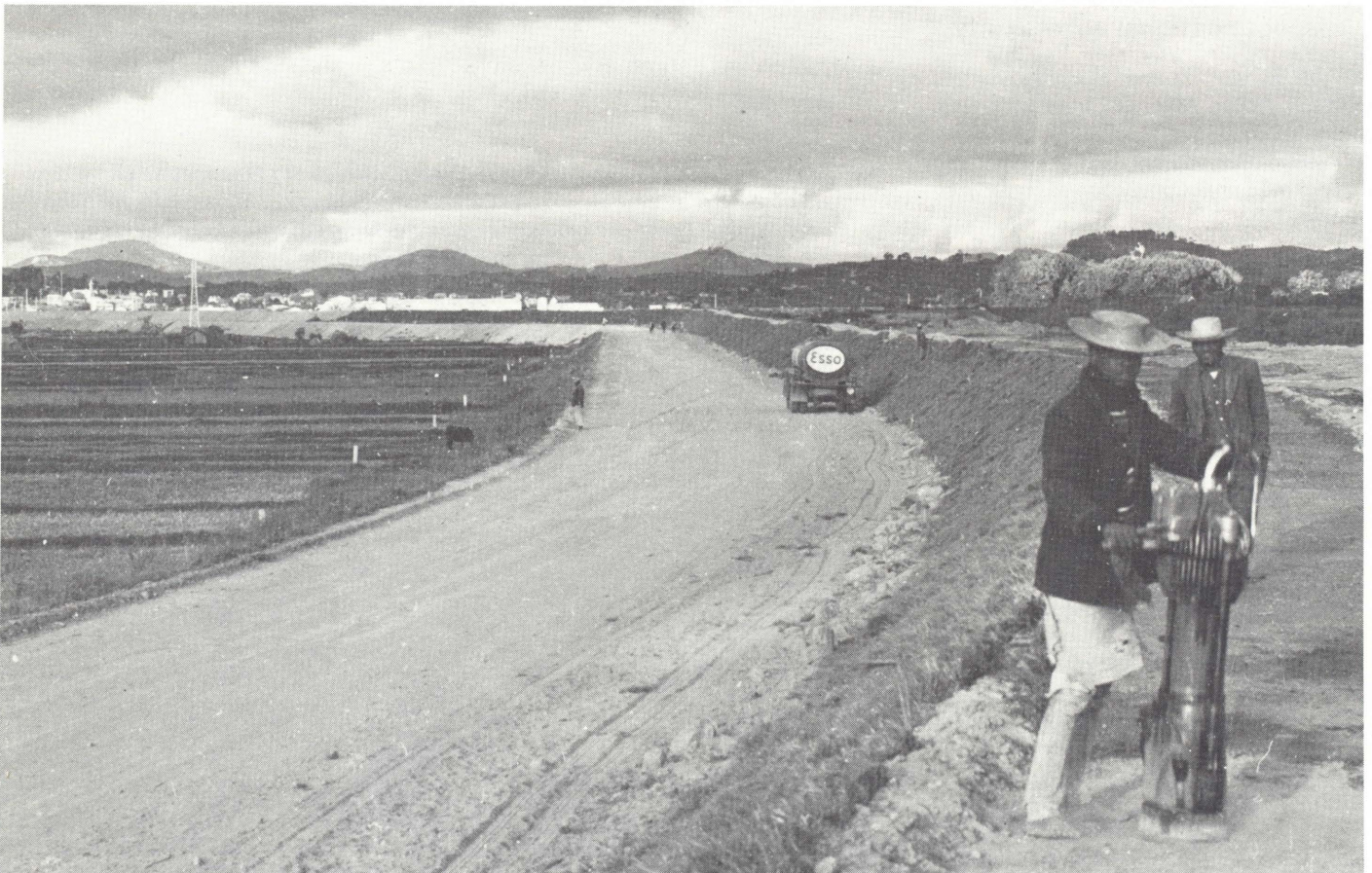
Flood wall on the river Ikopa
