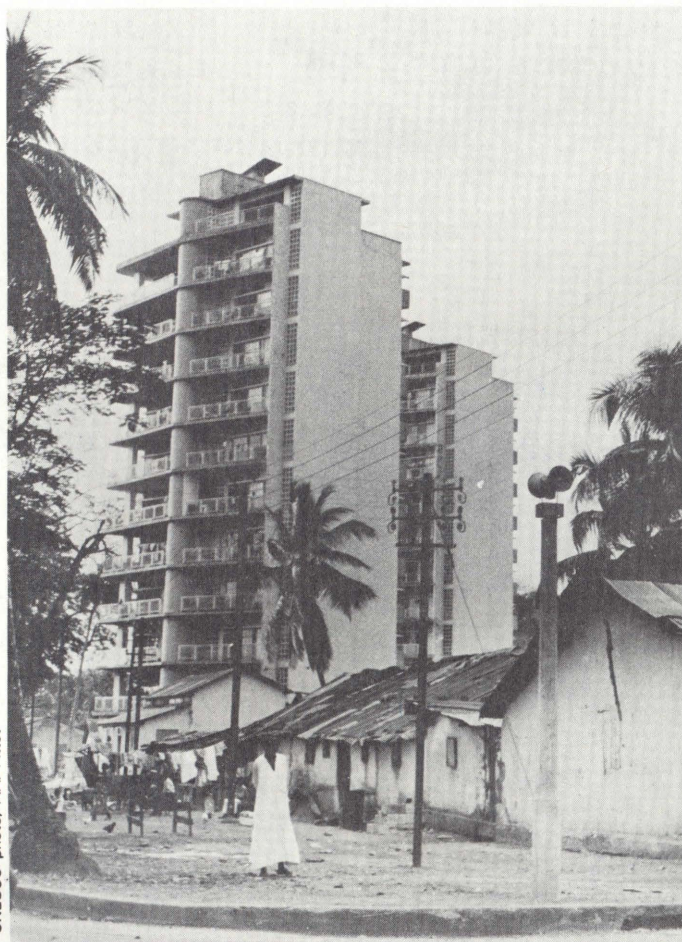
Tower blocks overshadow old houses in Conakry (Guinea)
