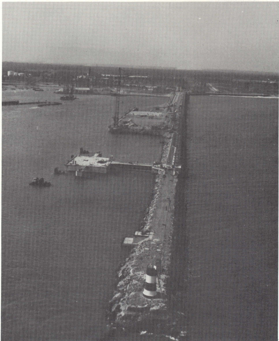
The main jetty
