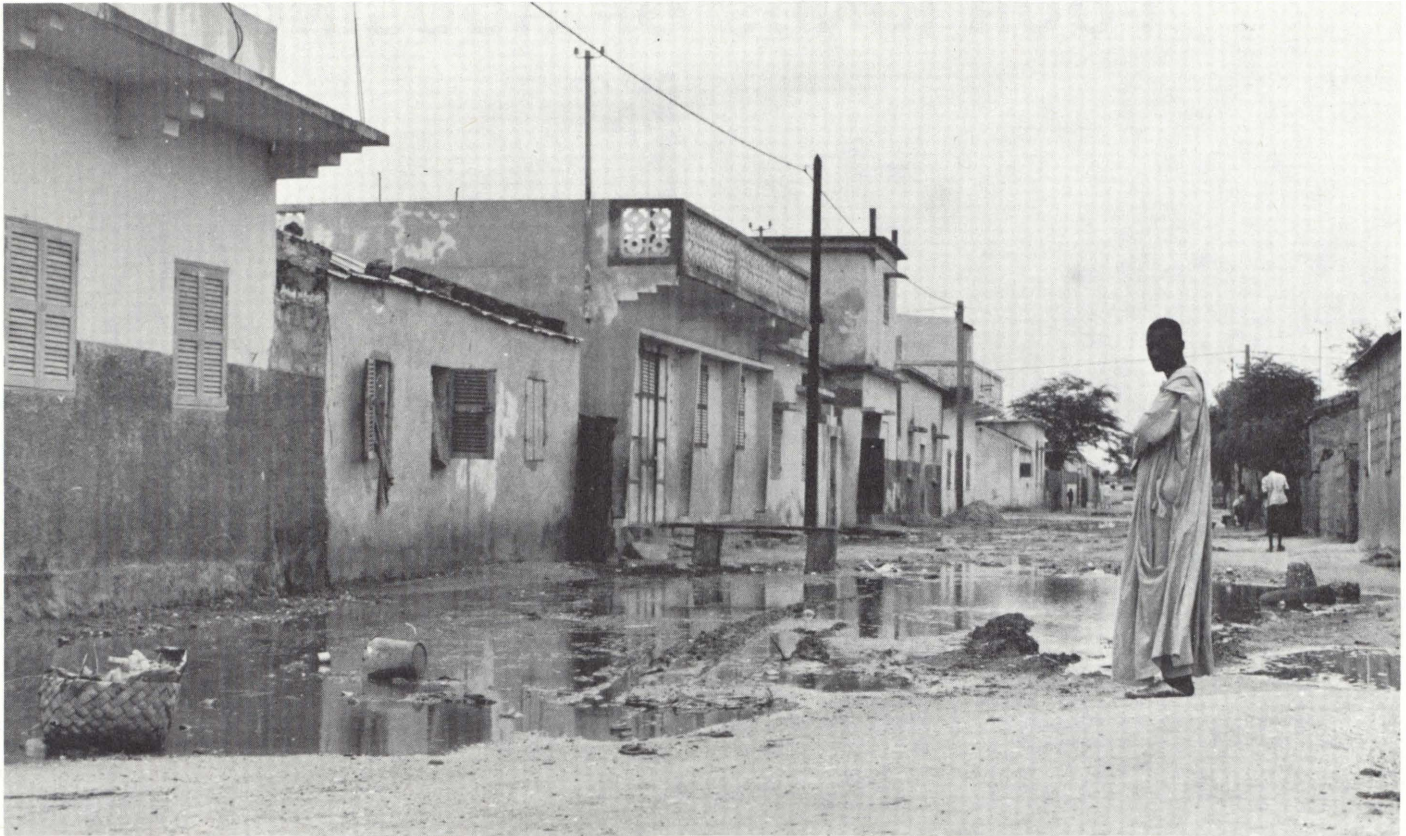
The result of inadequate drainage
