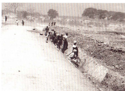
Food-for-work programme - Road construction.
