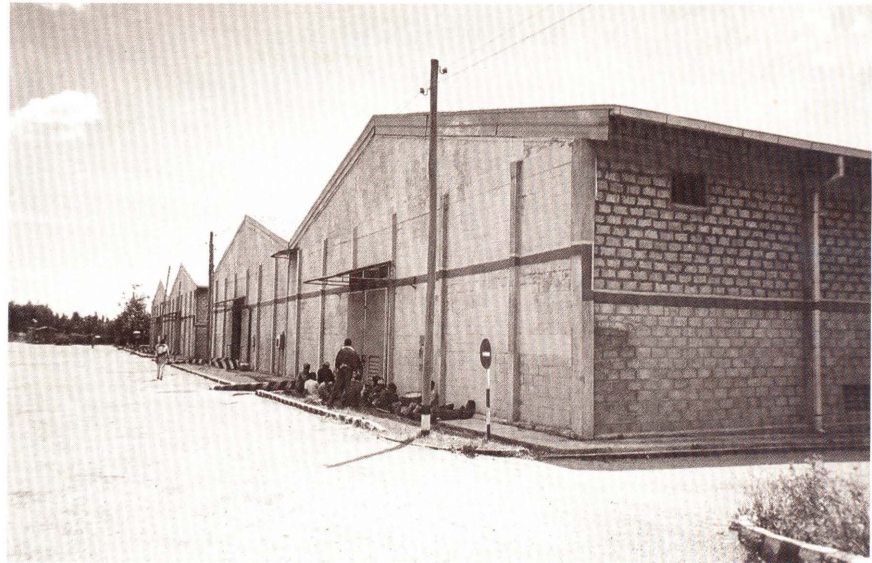
Storage hangar in Shashmane for the local purchase operation (Ethiopia).
