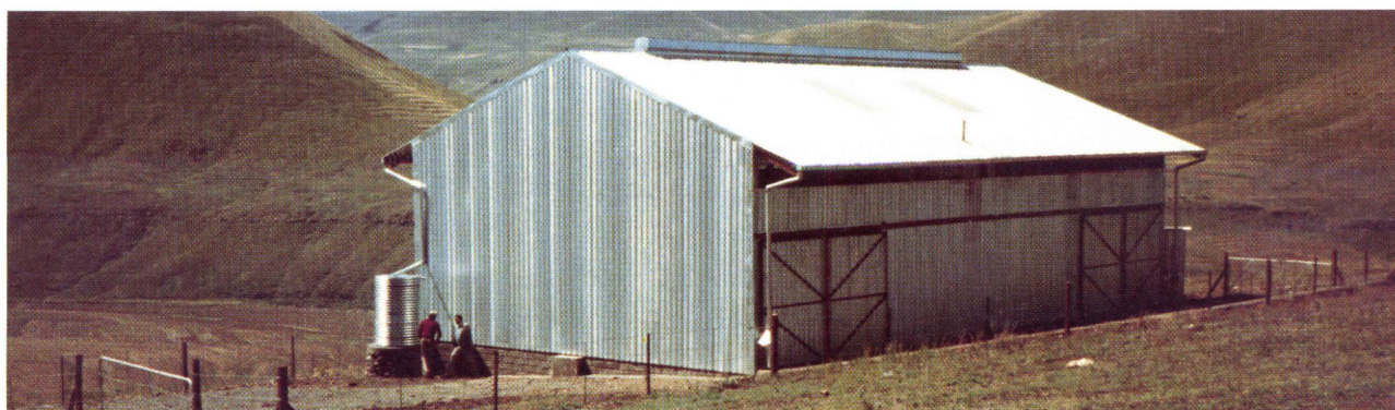
Cereal warehouse - Its construction was financed with counterpart funds (Lesotho).
