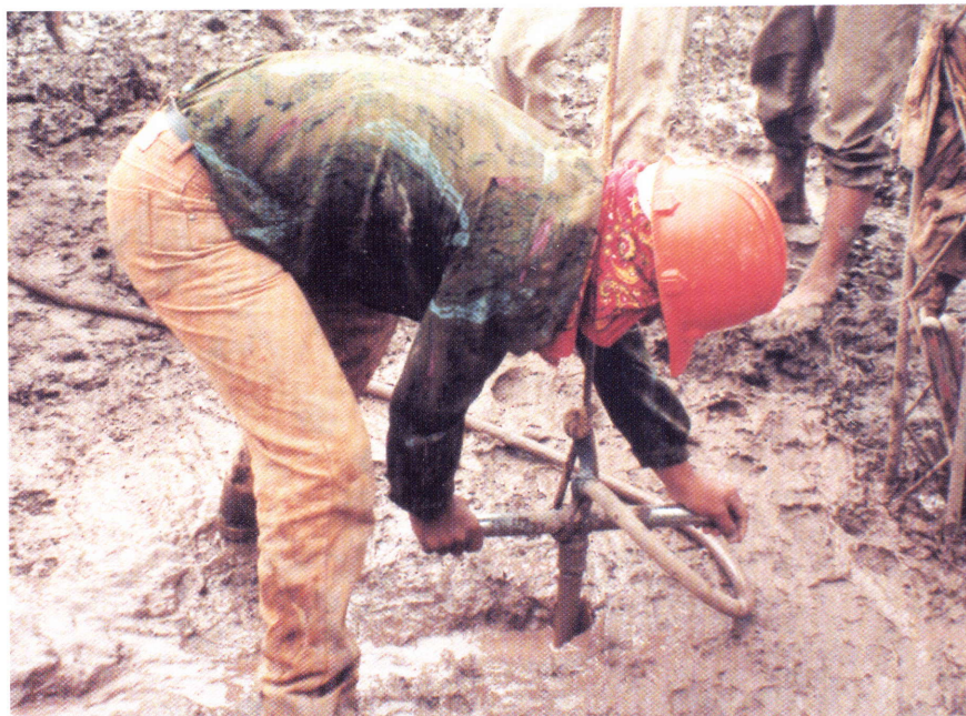
A man boring a potable water well in a field near the El Salvador-Honduras border zone.
