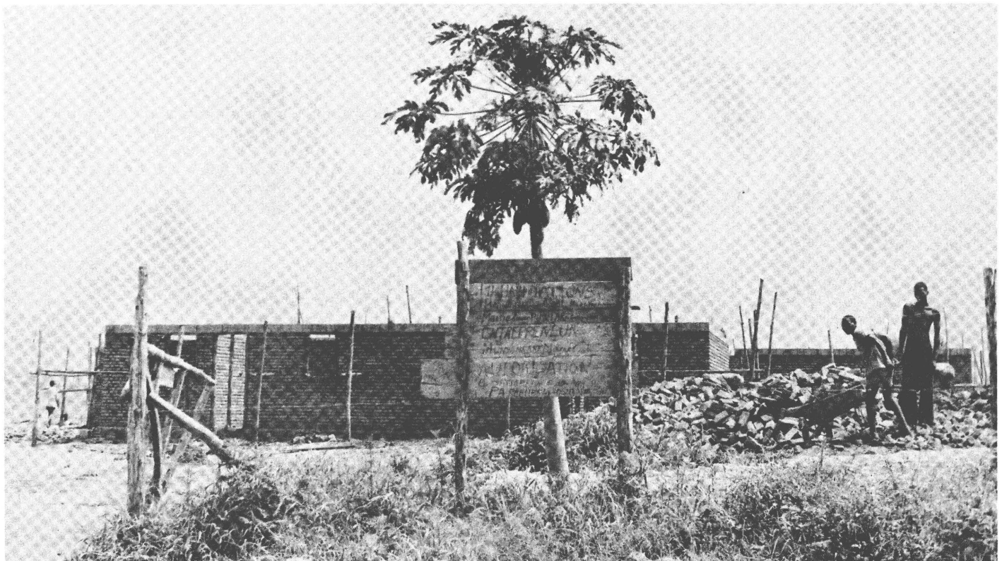
Housing for the handicapped in Mali, a joint EEC-NGO project
