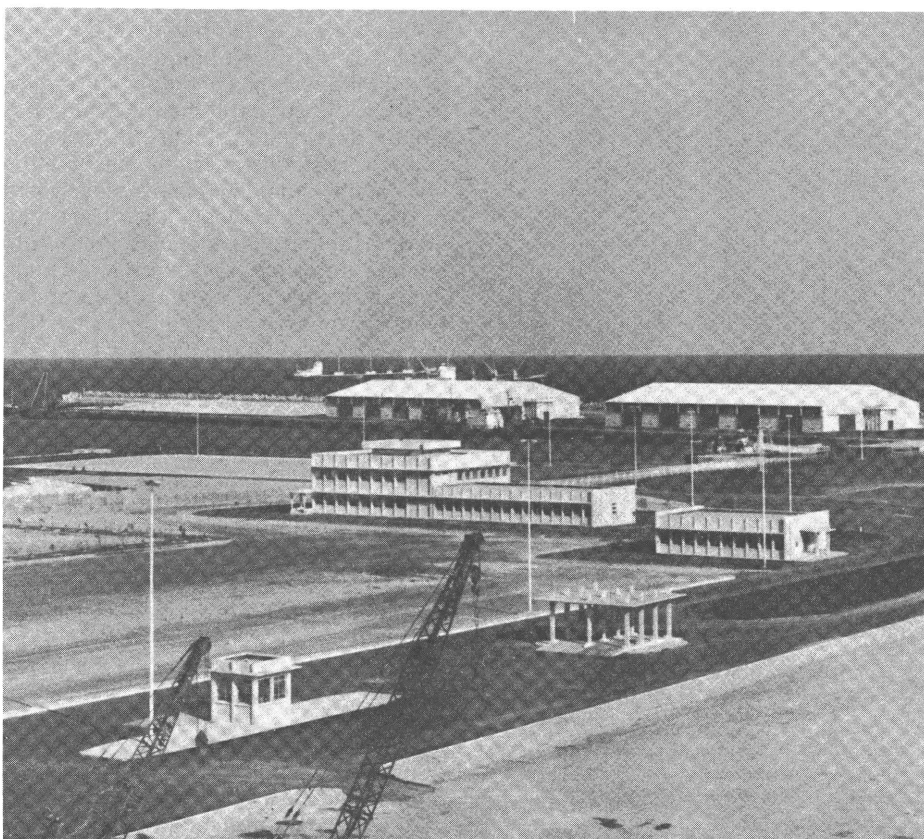
Italian construction firms have a long experience of development projects, such as this deep-water port in Mogadishu (Somalia)
