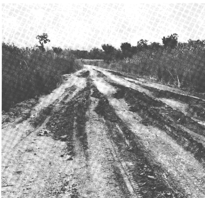
Too many sections of Africa's road network are little more than impassable tracks in the wet season
