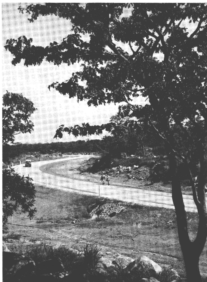
A good road linking two countries is not enough in itself to generate traffic immediately
