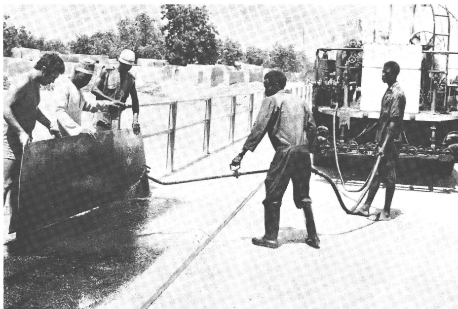
Spraying tar on pavements at Tessaoua
