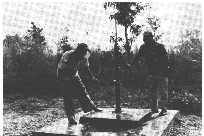
One of the 11 wells drilled during the project, to tap water 70 feet down
