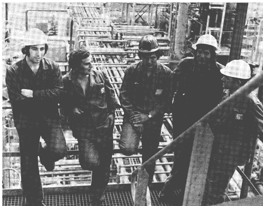
Construction and other manual and sometimes menial jobs are often taken by foreign workers
