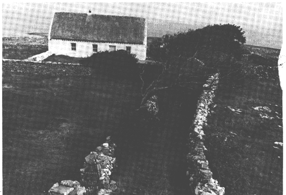
Traditional Irish cottage in the Aran Islands—just as much a part of the Community as the office blocks of the EEC capitals
