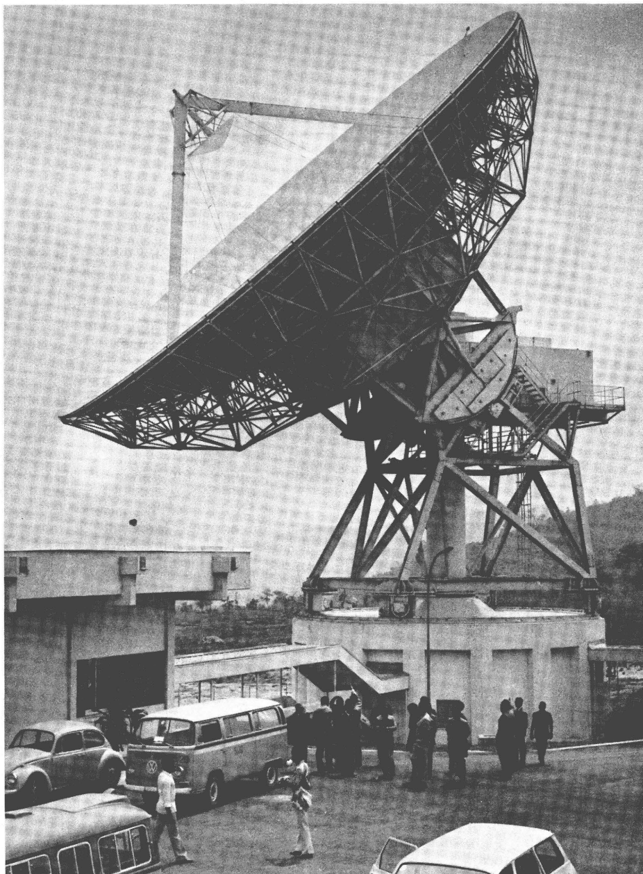
N'sele satellite telecommunication station, Zaire
