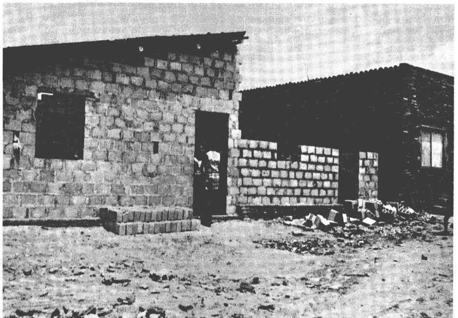
A house constructed from PATAC blocks nearing completion
