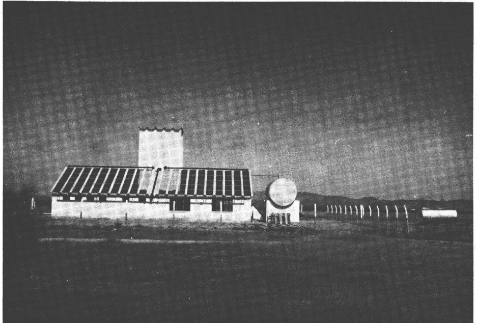
Solar-powered pump in Mexico
