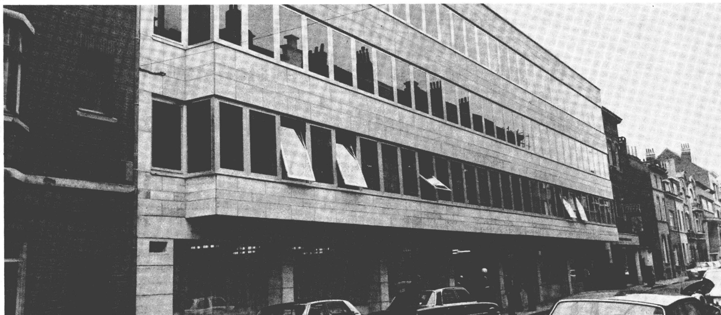
ACP House where the CDI has its offices
