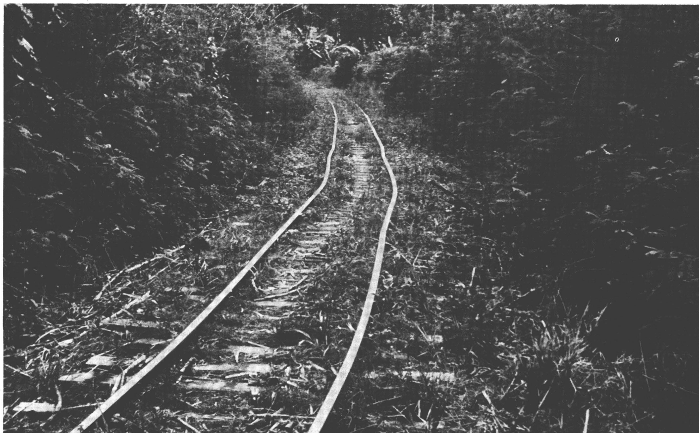
An African single track railway line. What volume of traffic can it handle?
