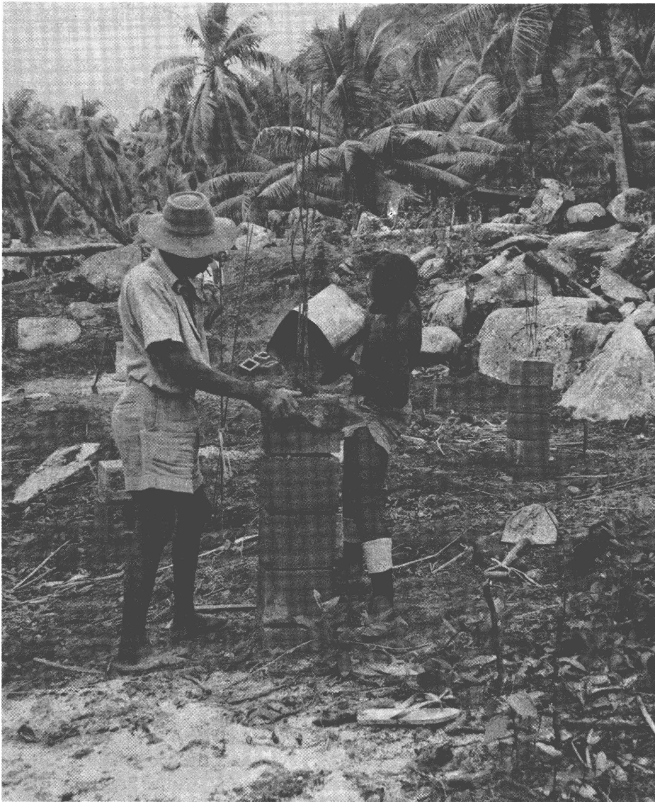
Starting to build a Seychelles house
