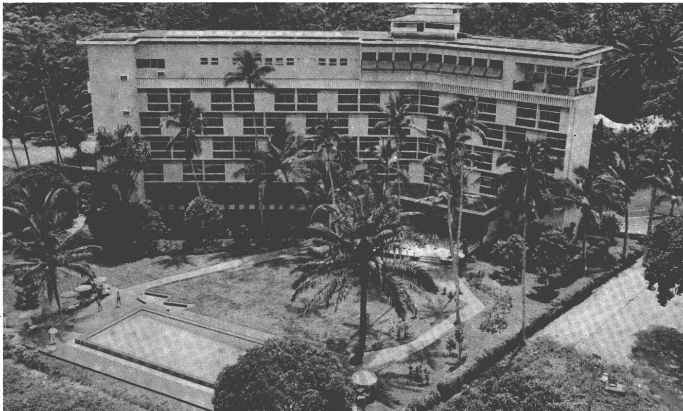
European capital has helped finance the reconstruction of the Hotel des Cocotiers in Douala
