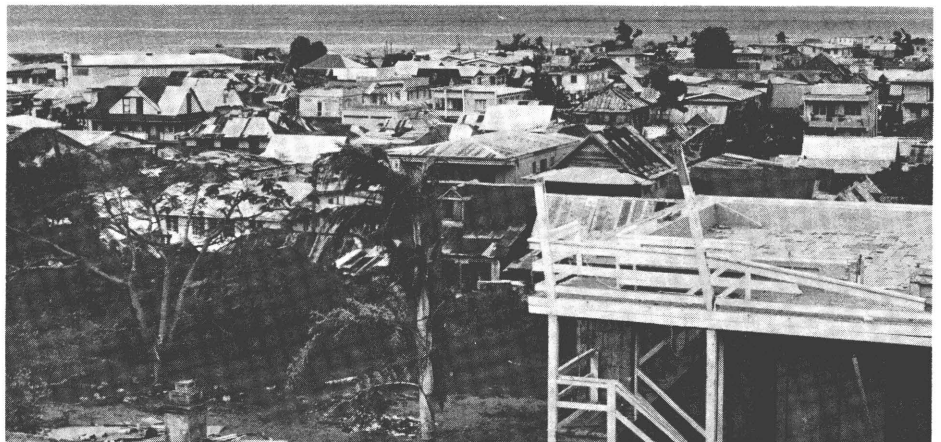
Six months later re-roofing is well in hand in Roseau, with the EEC providing 491 tonnes of roofing sheets
