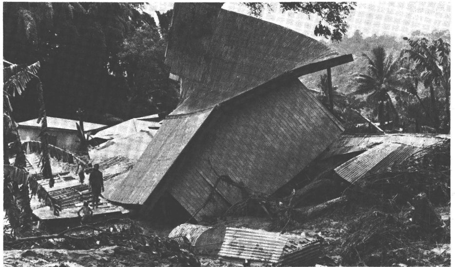
Thousands of buildings such as this school were destroyed by hurricane "Wally"
