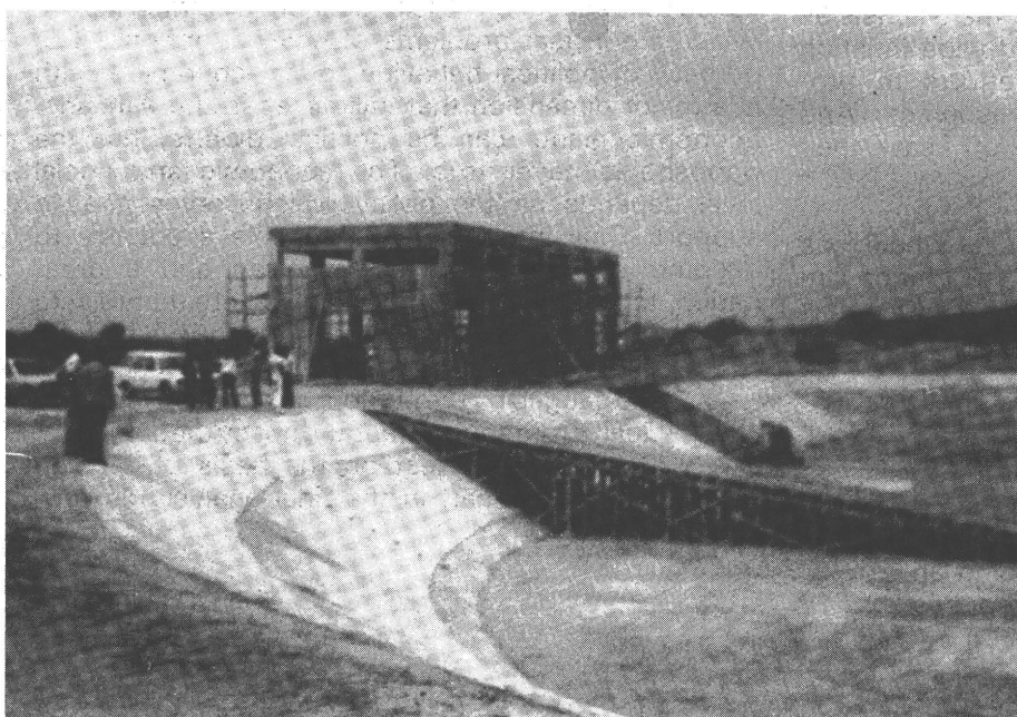
The second pumping station with its adjoining reservoir
