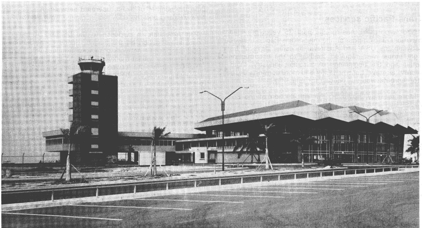
The Netherlands Antilles are the principal beneficiary of EEC aid in the field of air transport: photo shows the airport terminal building at Aruba, an EDF project
