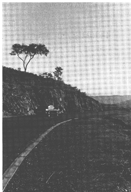
A partial view of the Blantyre-Chikwawa road, which was reconstructed with EDF aid; transport is of vital importance for landlocked Malawi
