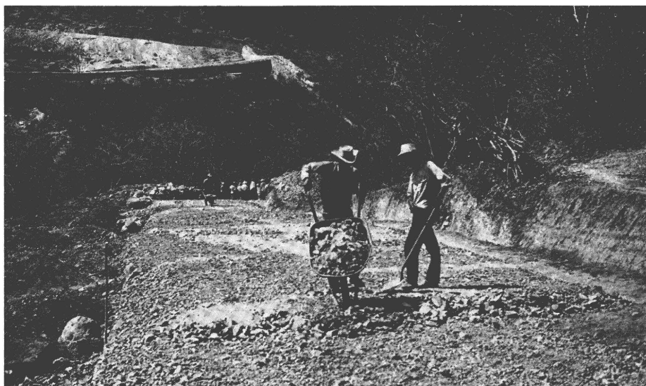
Labour-intensive road construction in Honduras
